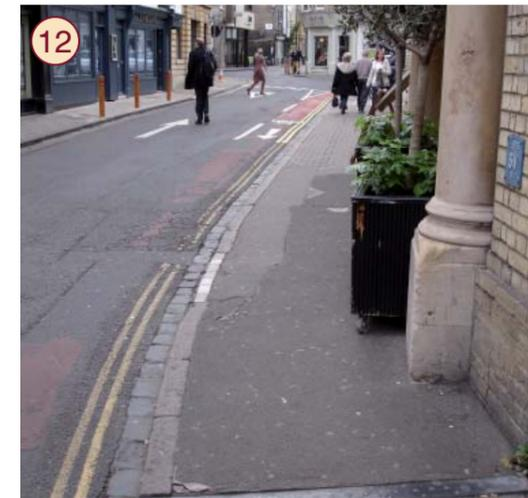
12 Pavements behind Guildhall very difficult for those in wheelchairs - narrow, steeply cambered and with few dropped crossings. Obstructed by planters and apparently randomly placed wooden bollards
